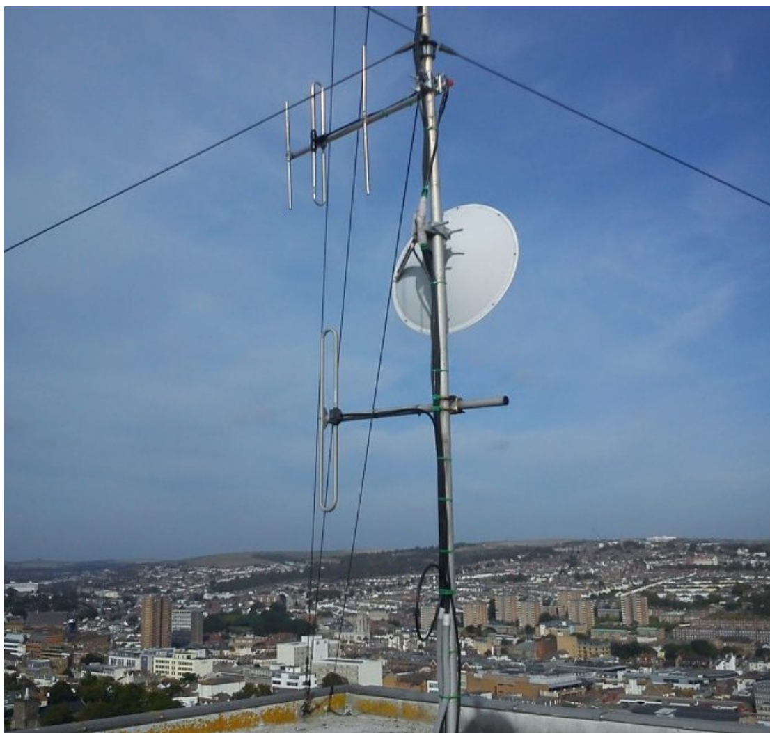
Fig 2: The three element Yagi mounted at a height of 4.4 m on the mast. The parabolic dish provided a reliable 1km IP link over Wi-Fi (100mW ERP).
